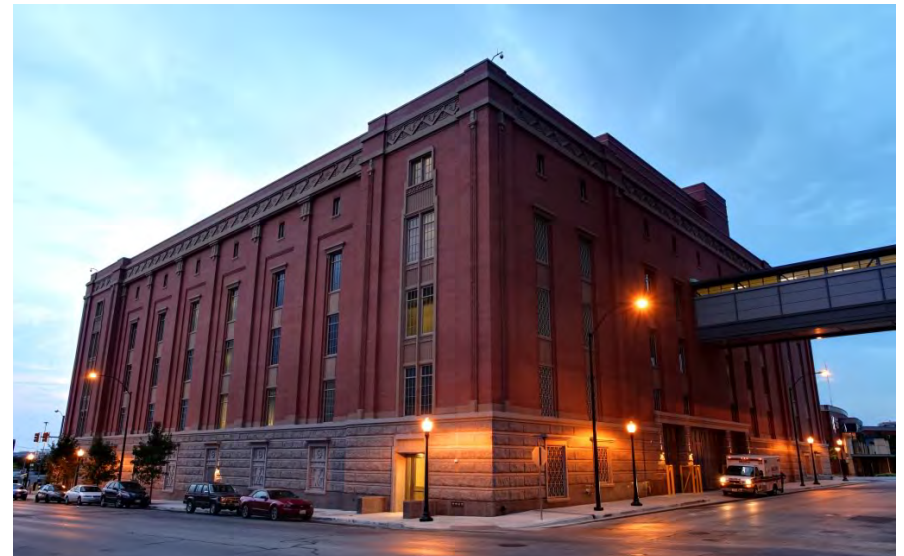
This skywalk is appropriate because it connects two correctional facilities.
