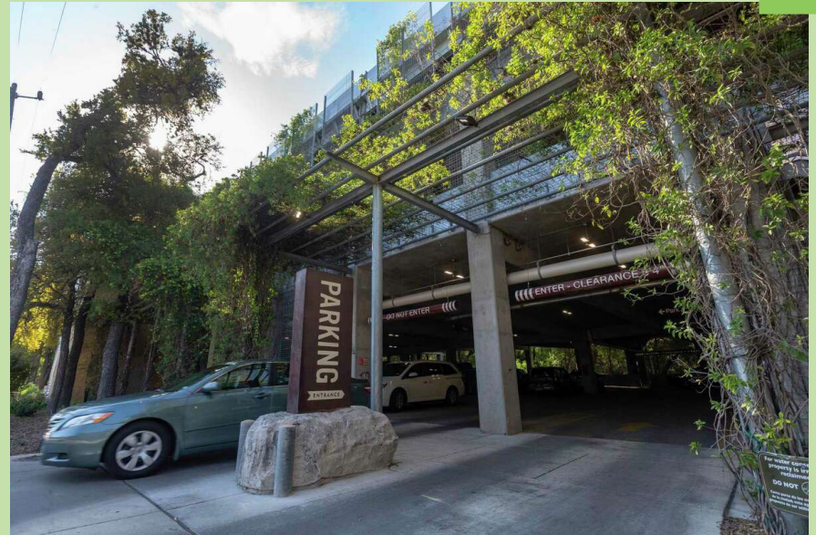
Green infrastructure: The parking garage of the Witte Museum (San Antonio, TX) incorporates sustainable measures such as a green living wall to reduce heat island effect.
